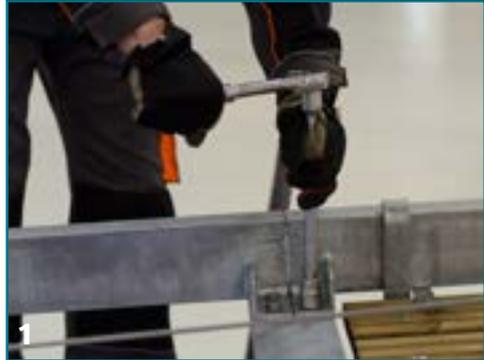
Use the supplied installation guideline in order to obtain 563 mm (22.17 in) as the distance between the rails (picture 2).
